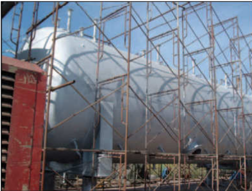
TSA on a process vessel
